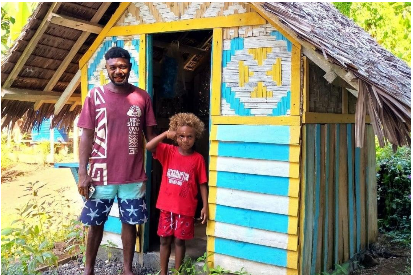
On the island of Vanualava, Kaltonga and his son are thrilled with a new Ventilation Improved Pit (VIP) toilet, a much-needed addition to community health and hygiene (© ABM AID 2026 / Terry Russell)
