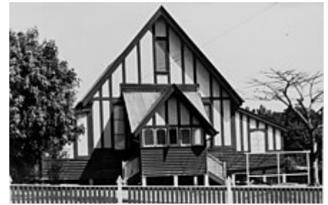
Figure 1: St Thomas Parish Hall c. 1940
