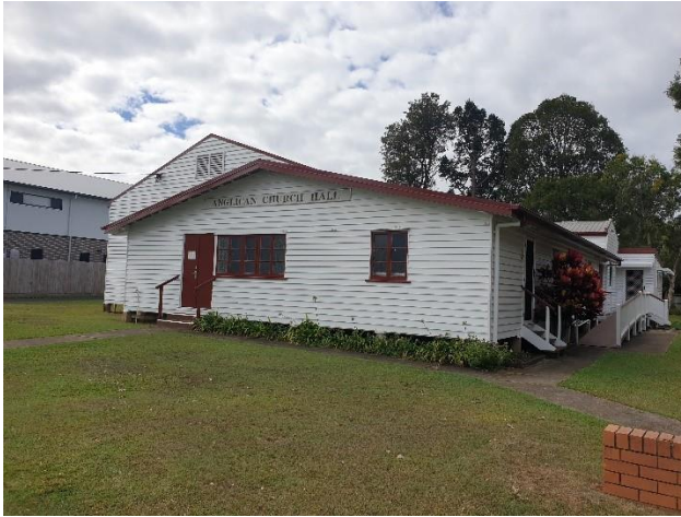
Banyo Parish Hall
